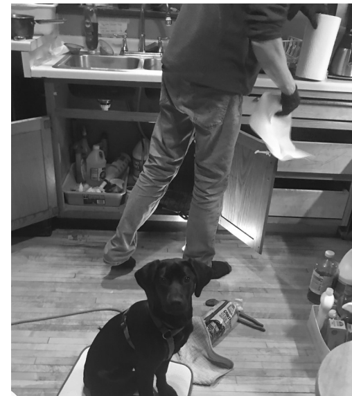
Mowgli supervises while Drew repairs the Olive Branch kitchen sink.
