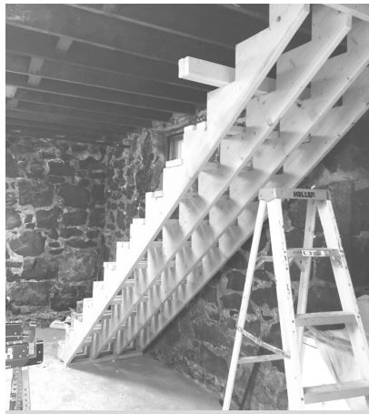
Construction of the Dorothy Day House basement stairs.
